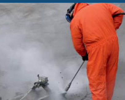
Removing concrete
