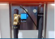
Solenoid valve for water supply
